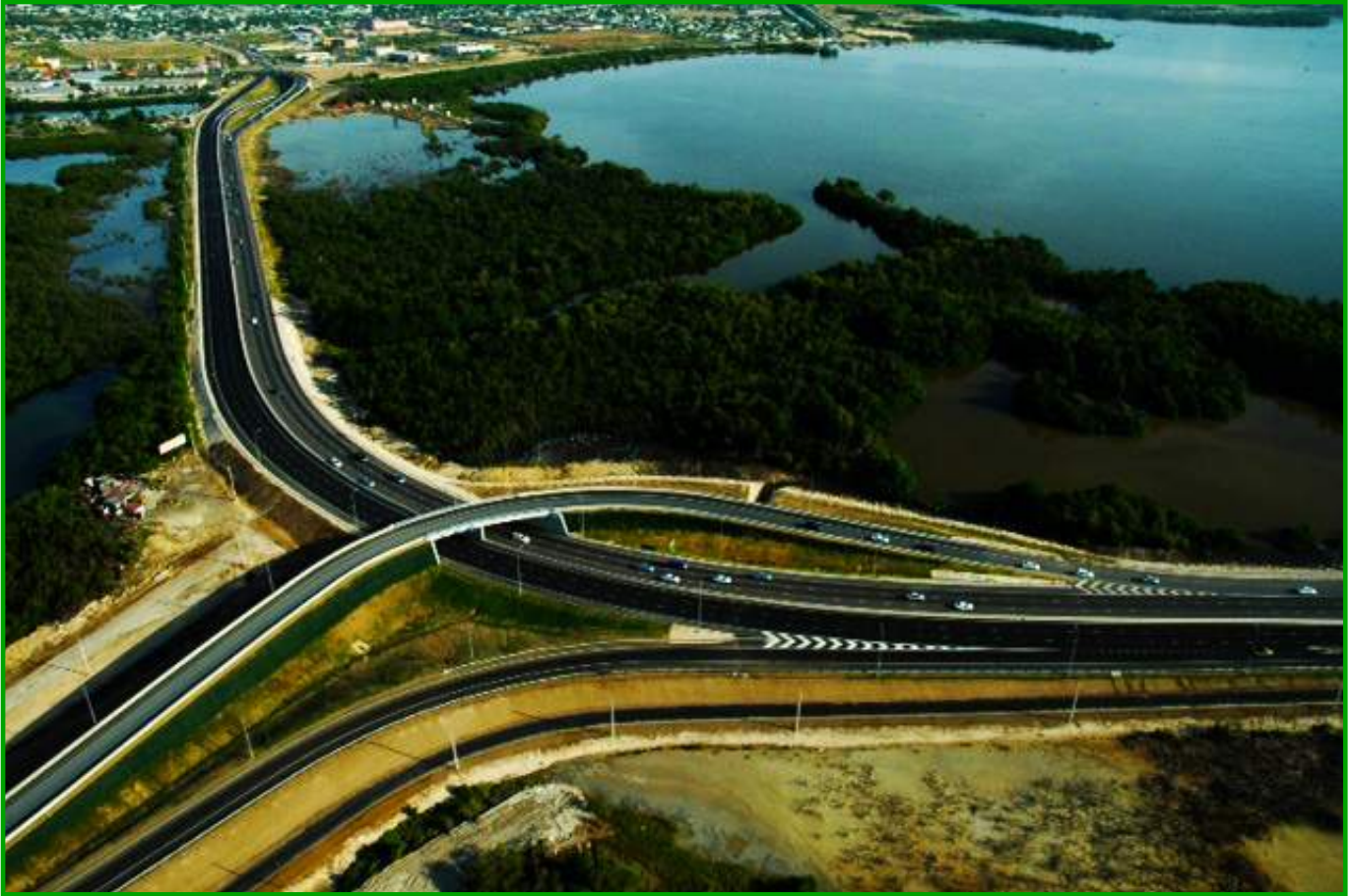
An aerial view of the Portmore toll road.
