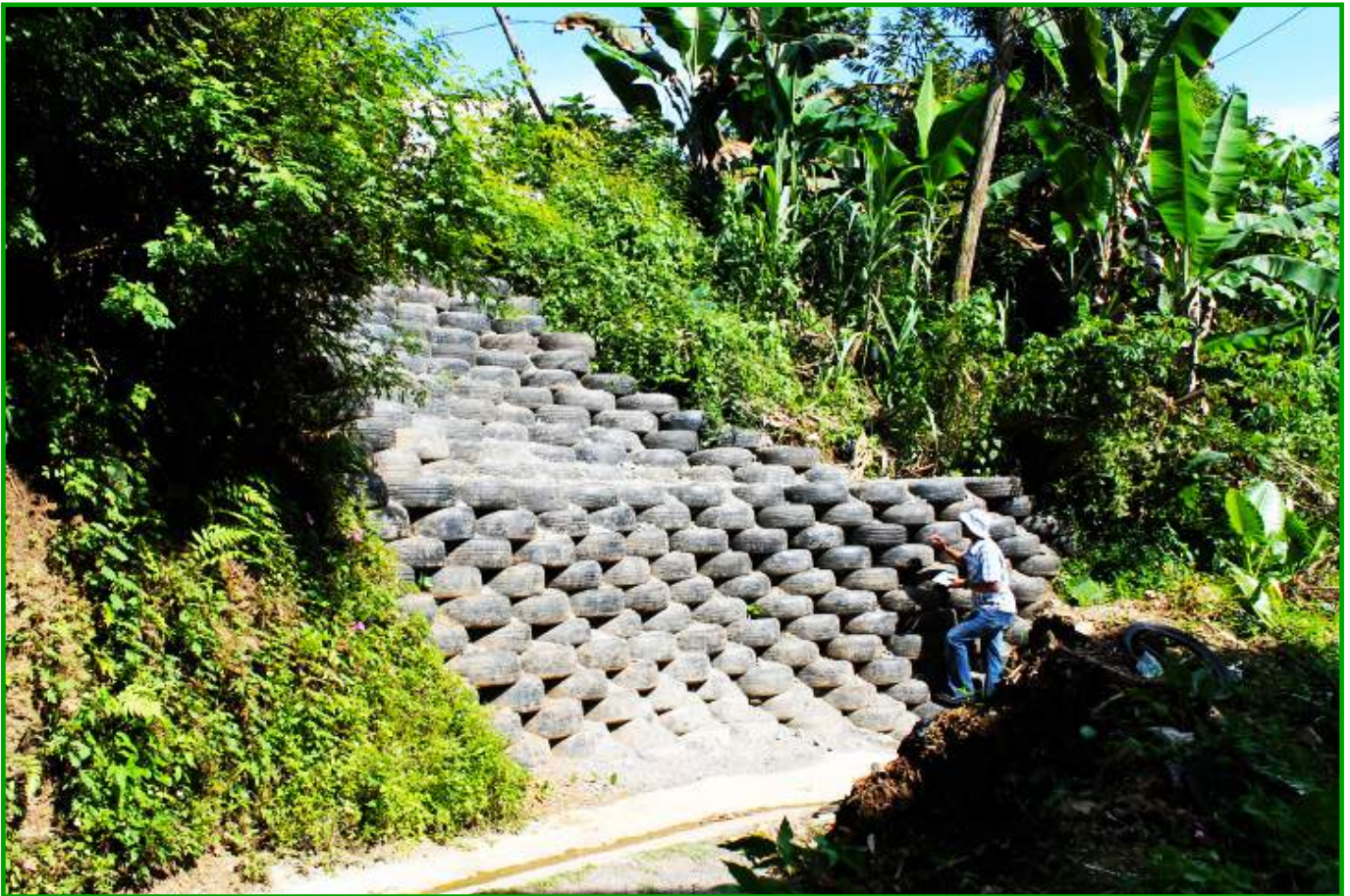
Tyre Soil Wall to reduce landslide risk in Breastworks, Portland.
